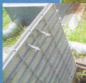
Aeration Tank Manhole Cover – JPP
