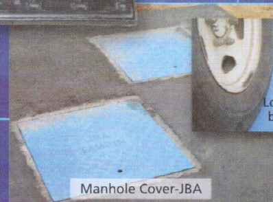
Drain Cover with FRP frame & Hinges
